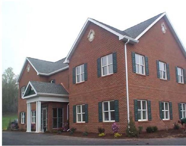
Almost ready for occupancy - the beautiful Conewago Place expansion in Hummelstown, PA
